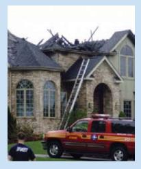
Direct strikes to buildings will commonly result in a fire that starts on the roof or in the attic. In this photo a brick home received a direct lightning strike to the roof resulting in a fire that caused \$600,000 in damage.
