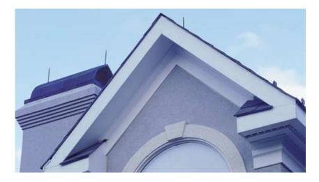
A lightning protection system is intended to last the life of the structure it protects and typically only requires maintenance if a home is changed structurally or mechanically. Such changes might include a new roof, an addition, a new electrical service or the installation of a satellite dish.
